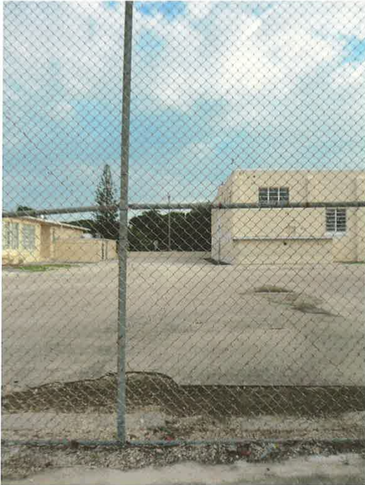
View of enclosed Whalton Street from United Street
