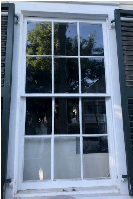
Double-Hung true divided-lite wood window
