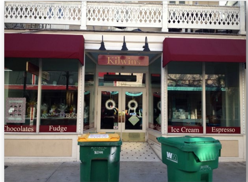
DESCRIPTIVE SIGNS CAN ONLY BE INSTALLED ON WINDOWS AND DOORS AND CANNOT EXCEED 20% OF EACH WINDOW OR DOOR GLASS PANELS.
