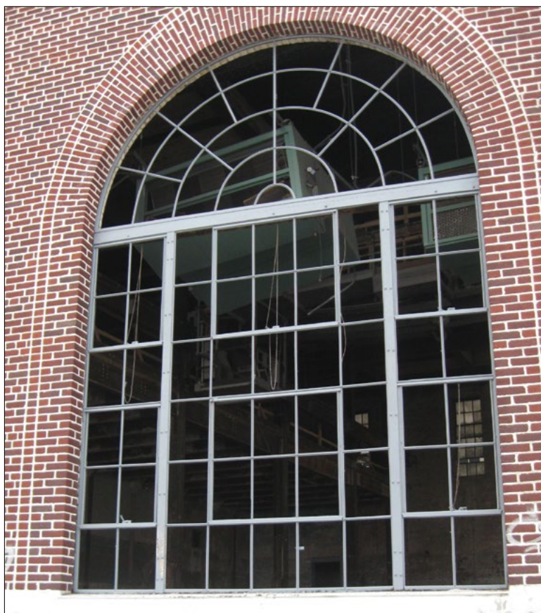
[12] This historic steel window has been cleaned, repaired, and primed in preparation for painting and reglazing.
